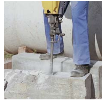
Breaking concrete
