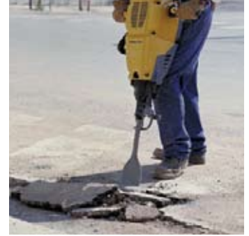
Cutting asphalt
